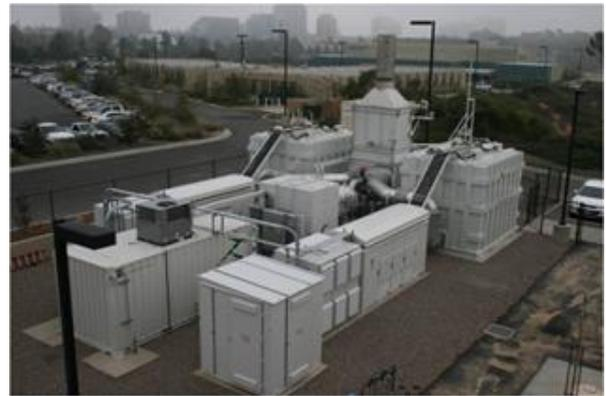
*2.8MW fuel cell power plant using FuelCell Energy's DFC3000 units*
