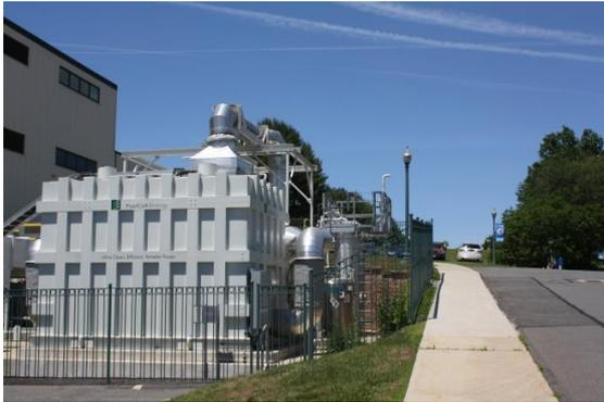
*FuelCell Energy's Direct FuelCell® electricity generation plant*
